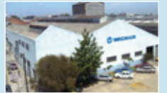
Plant in Buenos Aires, Argentina
