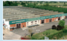
Plant in Palencia, Spain
