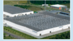
Plant in Gliwice, Poland
